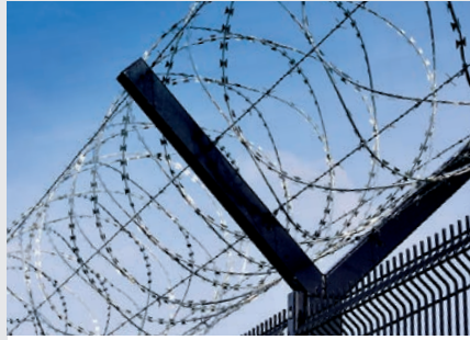
'Y' crank – 2 way crank at 45° to prevent climbing and increase security.
